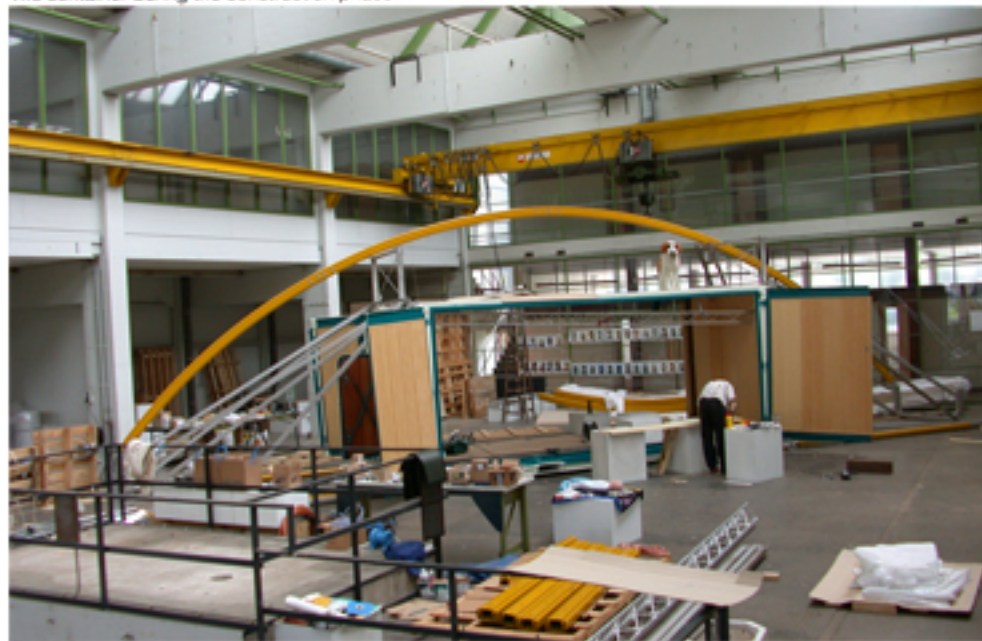
The container during the construction phase
