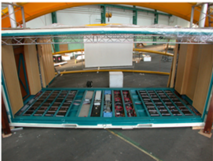
The ingenious power management system built into the container floor
